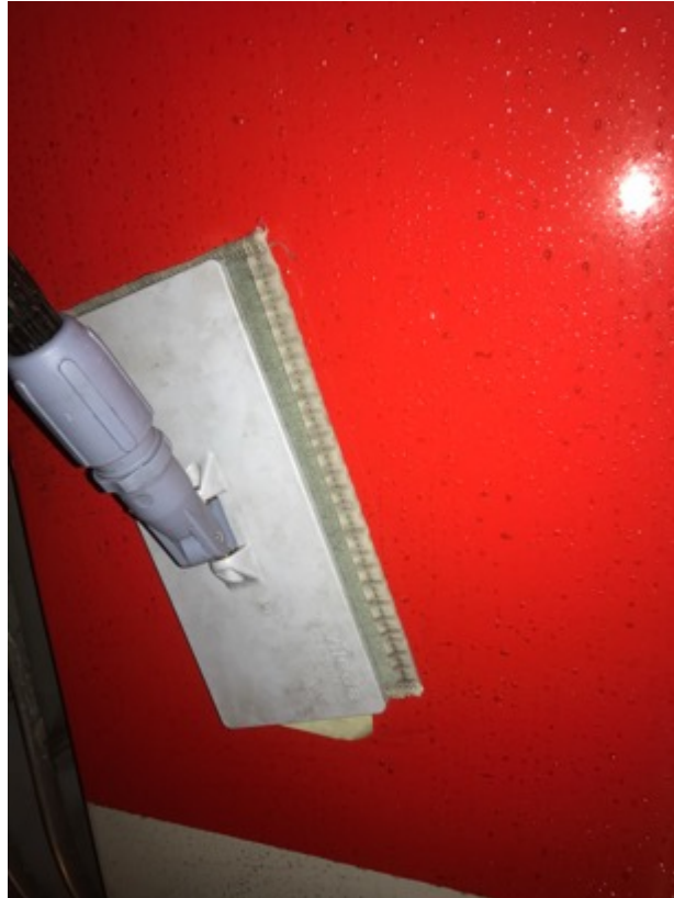
After wetting the surface with the cleaner leave up to 3 min. Observe a clear droplet formation.
